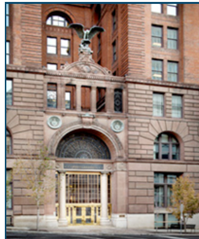
The scope of the project and the ultimate success in matching finishes with the original structure are demonstrated by this view of the building
