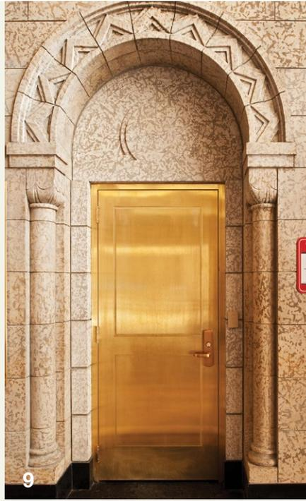
**“After” photograph of door to stairwell, etched and fire-rated**
