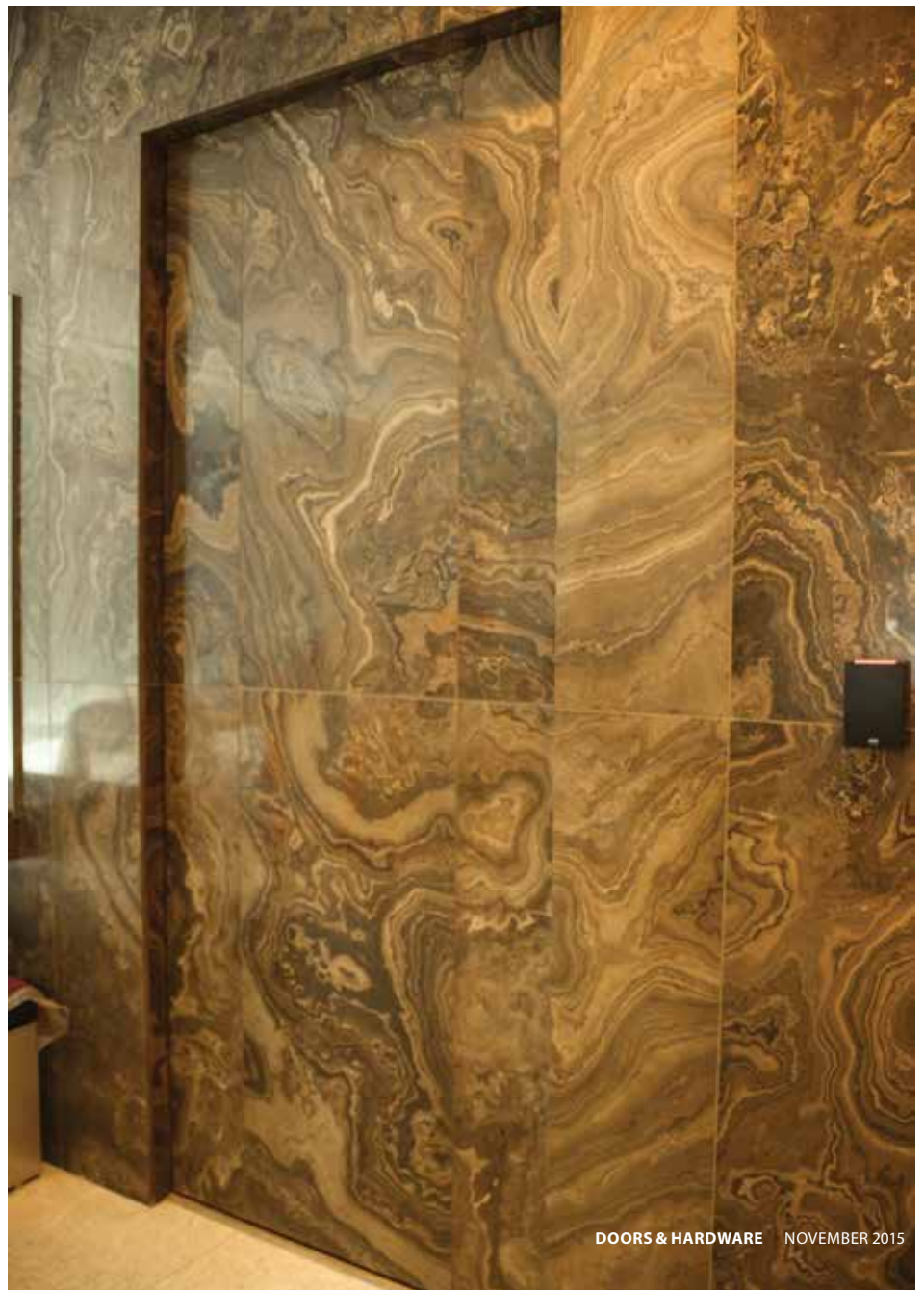
This stone-clad assembly ("push side" view) is card reader-operated and seamlessly assimilates to the surrounding wall.
