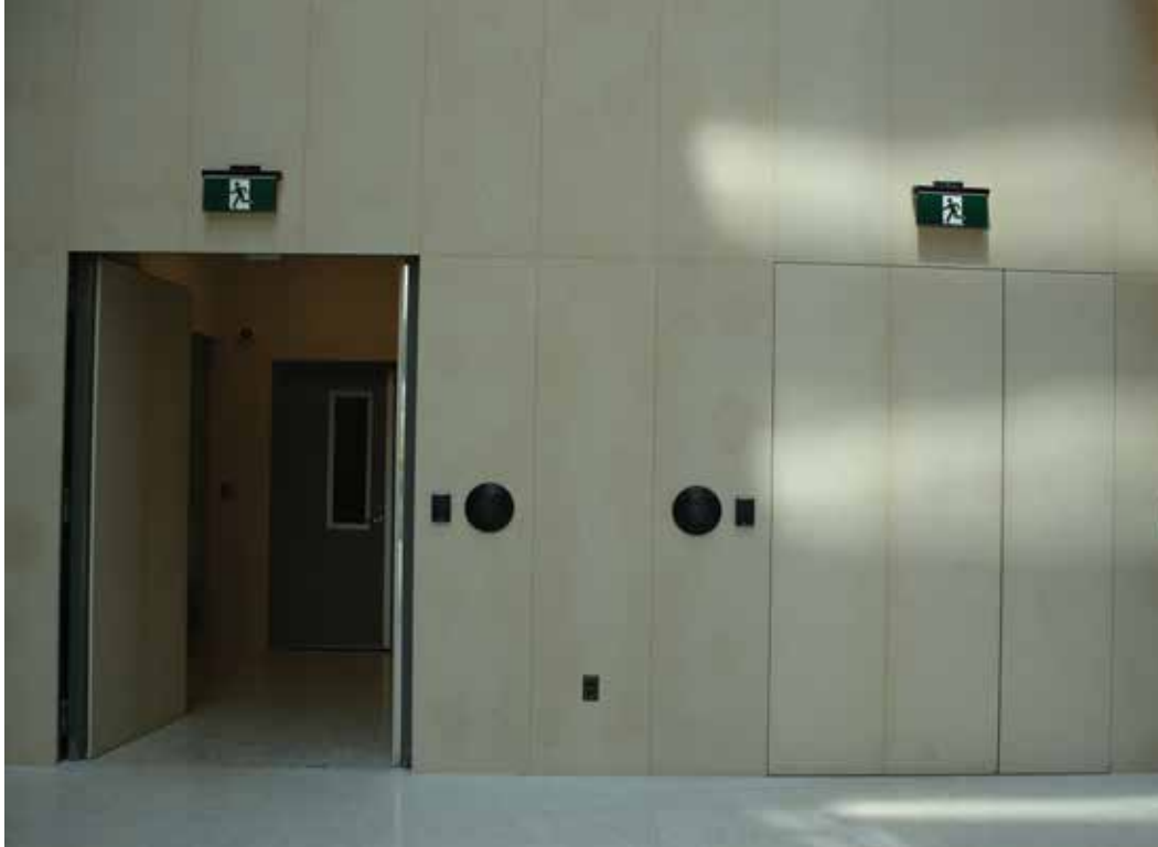
These acoustic door assemblies are slate-clad, designed to integrate with existing slate walls and are installed flush with the surrounding façade.
